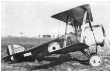
The precise identity of this aircraft is uncertain. It might have been the F.1/3 modified to production standard with three-piece upper wing and lengthened ailerons; alternatively it might have been a later prototype or an early production aircraft.
