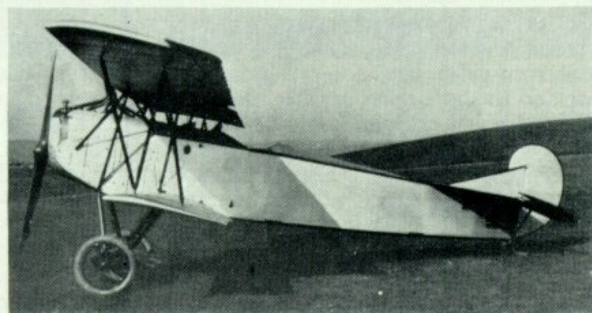
An experimental D VII fitted with "rhino horn" type manifold exhausting over the top wing. (Photo: Egon Krueger)
