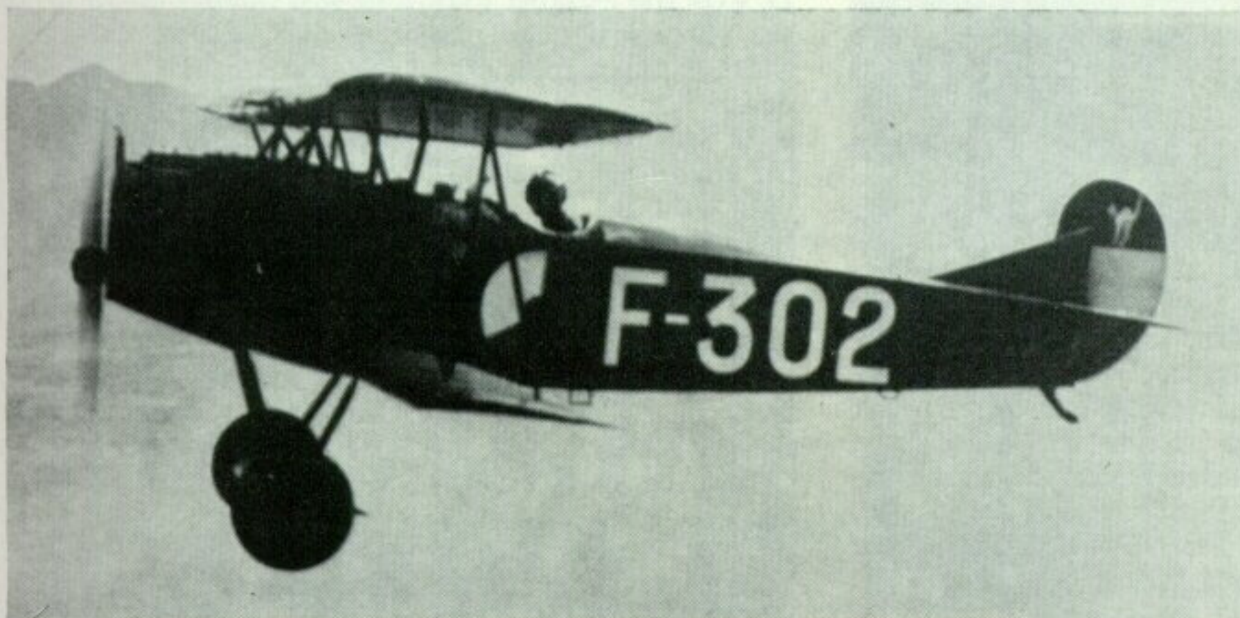
Fokker D VII (O.A.W.) 4197/18 of Jasta 78. Note patchwork painting of motor hood panels to simulate camouflage pattern. (Photo: Egon Krueger)
