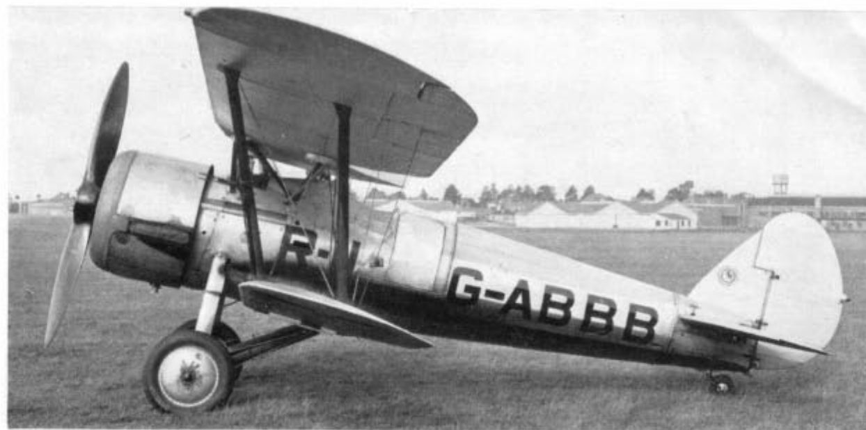
Bulldog 11A, G-ABBB, R-11, c/n 7446, with Aquila I engine in September 1935. Became K2227 in 1961 (see photo page 2). Originally with Gnome-Rhône 9ASB. Stored at Filton until 1939, when presented to Science Museum. Returned to Filton for reconditioning 1957; crashed 13th September 1964. Below: The original K2227 of No. 56 Squadron. Only two Bulldogs had this engine cowling—see side-view colour drawings on page 7. (Crown copyright)
