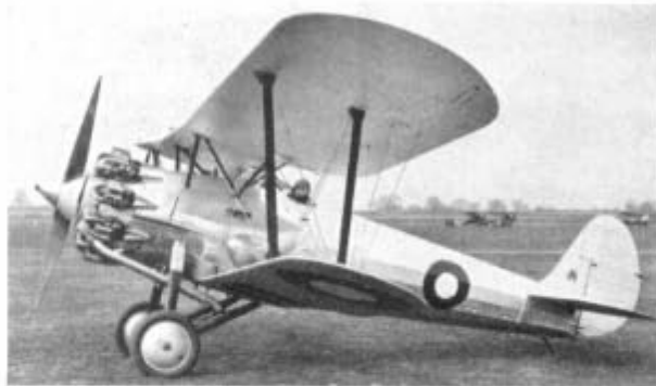
Left: Bulldog IIA, Danish Air Force. Note gun blister under cockpit and position of trough (0-300 Madsen m/gs). Right: Finnish Bulldog IVA, BU59, Mercury VIS.2 engine, similar to R-7, illustrated on a previous page.
