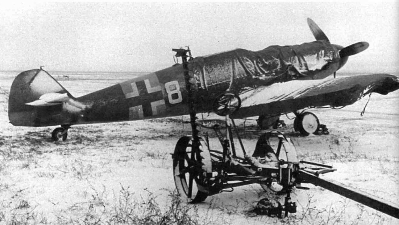
Above: A lot of manpower was required to clear the runways and taxiways after heavy falls of snow had paralysed Luftwaffe activity on most of its forward air strips during the hard winter of 1941-2. The lack of warm clothes for its mechanics, and of 'warm-up' systems for the aircraft, severely affected aircraft maintenance. Consequently serviceability fell as low as 30% in most units.
