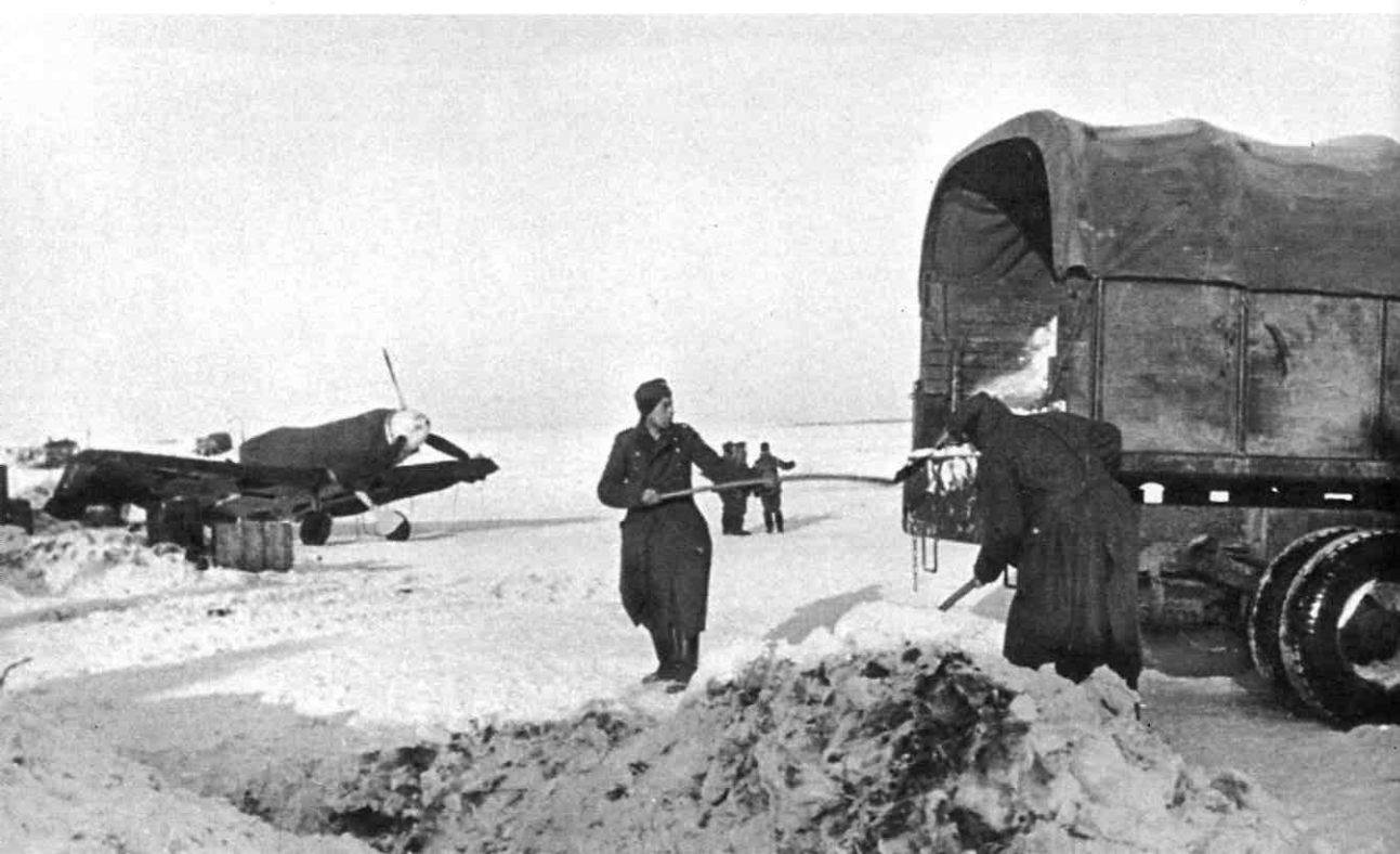
Above: A lot of manpower was required to clear the runways and taxiways after heavy falls of snow had paralysed Luftwaffe activity on most of its forward air strips during the hard winter of 1941-2. The lack of warm clothes for its mechanics, and of 'warm-up' systems for the aircraft, severely affected aircraft maintenance. Consequently serviceability fell as low as 30% in most units.
