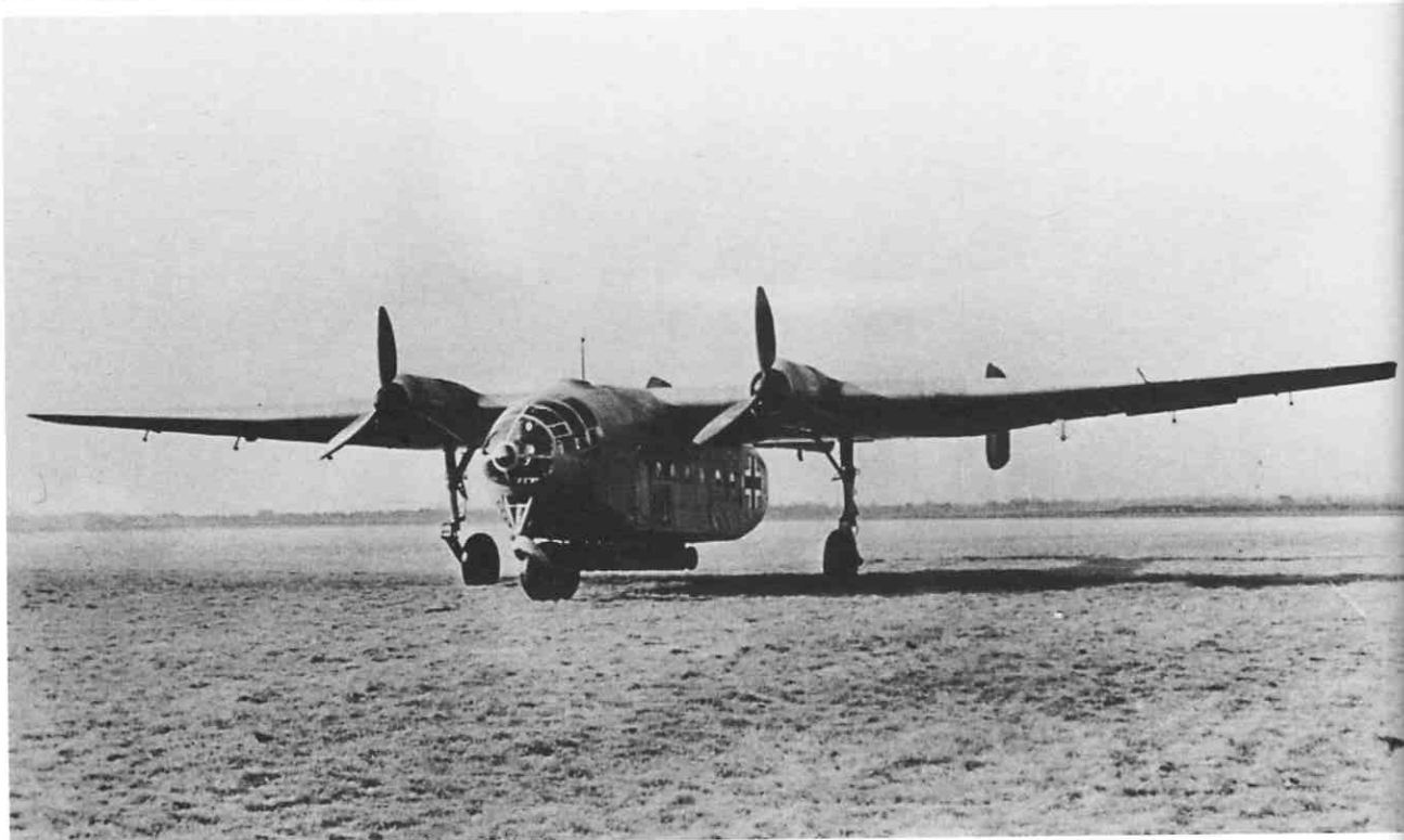
Above: The Arado Ar 232 was the forerunner of the modern military transport. The pod and boom configuration allowed rear loading through clamshell doors aft, while a multi-wheel undercarriage allowed it to 'squat' for loading. The first two prototypes, one of which is seen here under the designation of Ar 232A-0, were powered by two BMW 801A radial engines.
