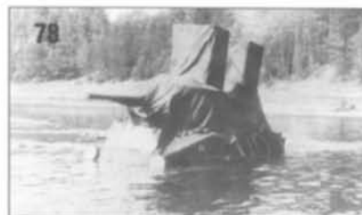
77,78. Испытания опытного танка подводного буксирования БТ-5ПБ. Август, 1934 г. The evaluations of the BT-5PB — the tank capable of submerged water crossin being towed by another vehicle. August 1934.
